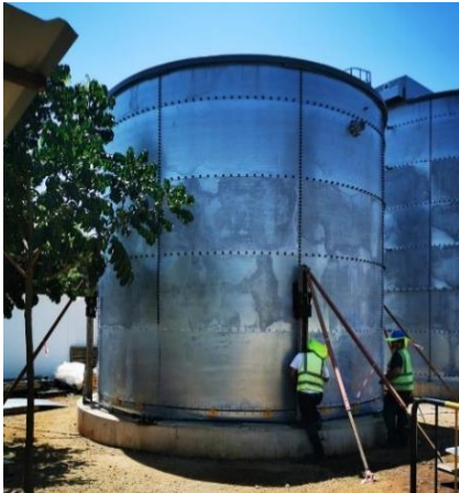
20. Installation of 4 th Ring
