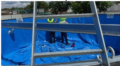
7. Liner Installation - 1 st Tank
