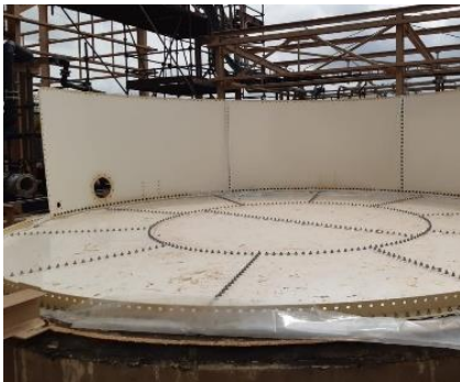
6. Installation of 1 st Tank Ring
