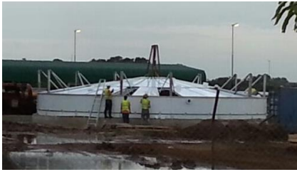
7. Installation of 1 st Ring
