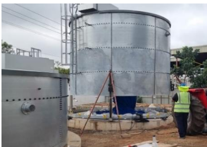
13. Installation of 4 th Ring - 2 nd Tank
