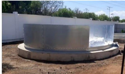
5. Installation of 6 th Ring - 1 st Tank
