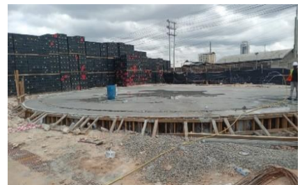
3. Slab Curing Process
