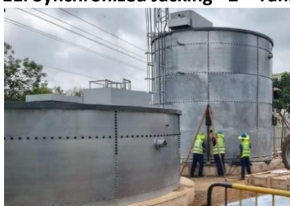
14. Installation of 3 rd Ring - 2 nd Tank
