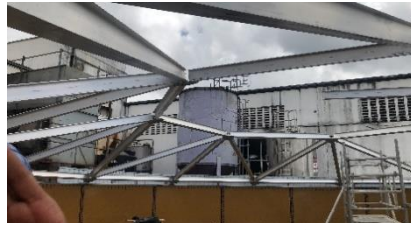
8. Geodesic Dome 1 st Ring
