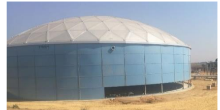
20. Installation of 4 th Tank Ring
