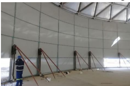
21. Installation of 5 th Tank Ring
