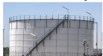
6. Spiral Staircase & Guard Rail
