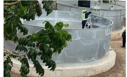
9. Installation of 7 th Ring
