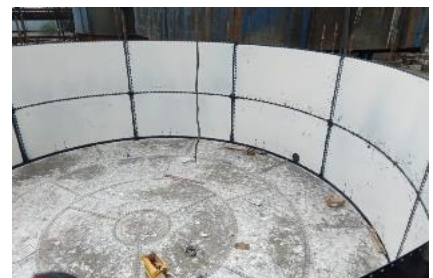
6. Installation of 2 nd Ring
