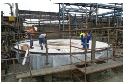
4. Steel Floor & Curb Angle
