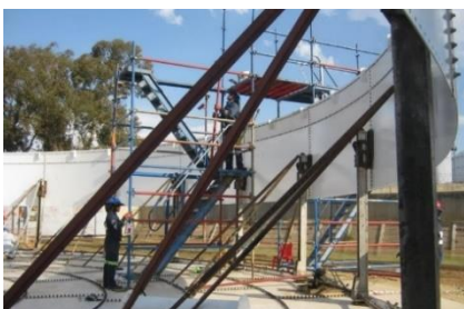
4. Synchronized Jacking
