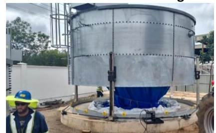
12. Installation of 5 th Ring - 2 nd Tank
