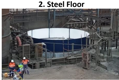
5. Installation of 1 st Ring
