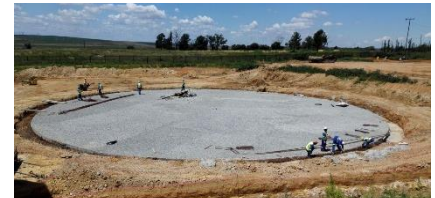
3. Concrete Slab
