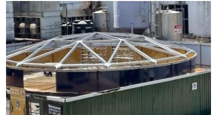
9. Geodesic Dome Framework
