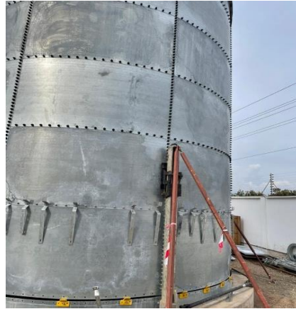
21. Installation of 2 nd Ring
