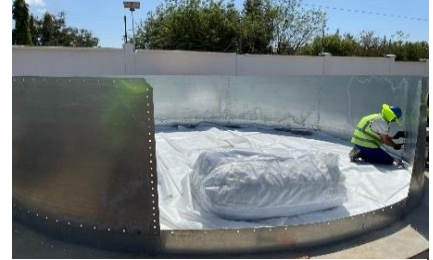
6. Installation of 7 th Ring - 1 st Tank
