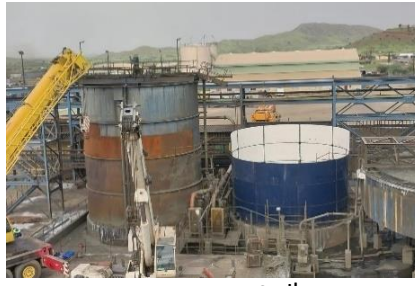
8. Installation of 4 th Ring
