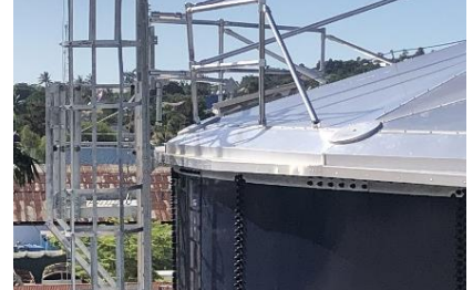
21. Partial Guardrail
