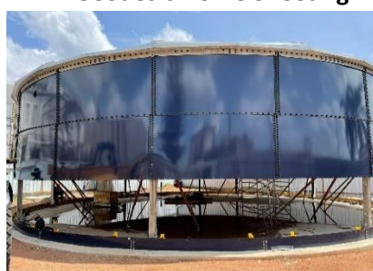
14. Installation of 2 nd Ring
