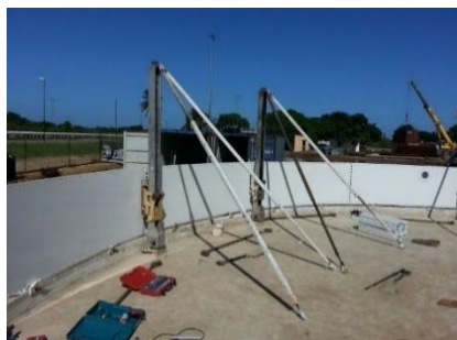
2. Synchronized Jacking
