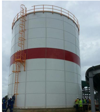
11. Installation of 7 th Ring
