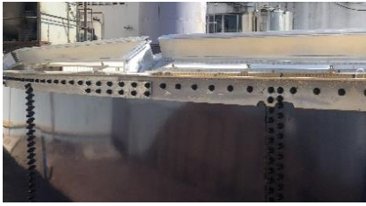
7. Geodesic Dome Footing
