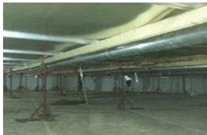
2. Completed IFR Bottom Section
