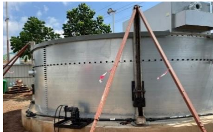
11. Synchronized Jacking - 2 nd Tank
