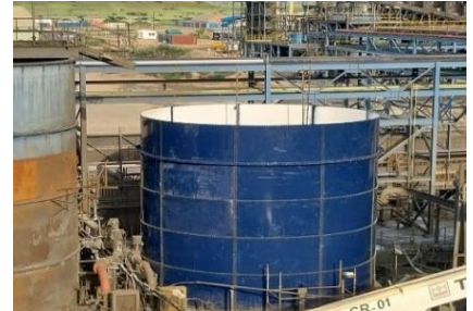
9. Installation of 5 th Ring
