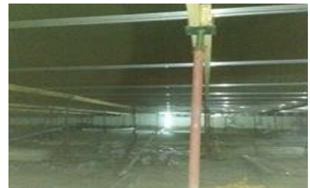
3. Completed IFR Bottom Section
