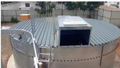
10. Roof Installation - 2 nd Tank
