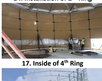
14. Installation of 2 nd Ring
