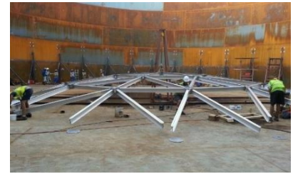
3. Installation of 1 st Dome Ring
