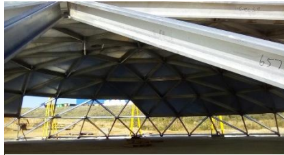
10. Erection of Dome with Quad Pods
