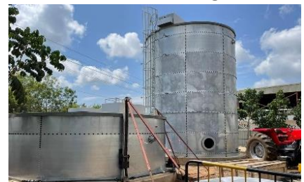
15. Synchronized Jacking - 1 st Tank
