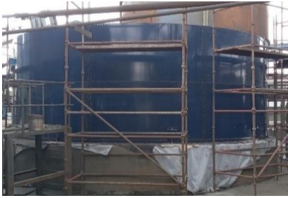
7. Installation of 3 rd Ring
