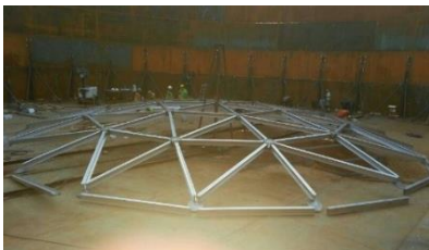
4. Installation of 2 nd Dome Ring
