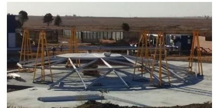
6. Installation of 2 nd Dome Ring
