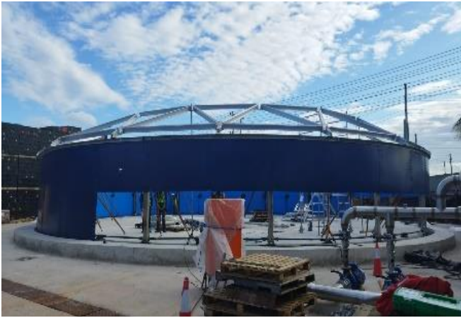
7. Installation of 2 nd Ring
