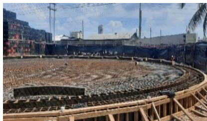
2. Steel Works for Slab
