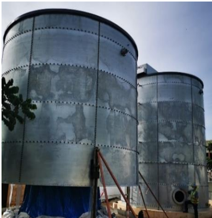
16. Installation of 2 nd Ring
