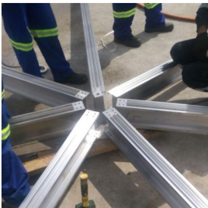
4. Apex Geodesic Dome
