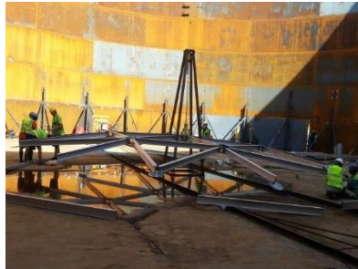
2. Installation of 1 st Dome Ring
