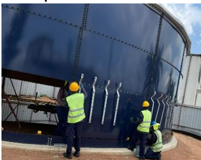
16. Wind Girders on the 3 rd Ring
