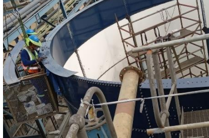
11. Eave Angle Installation
