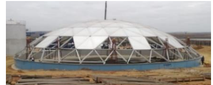
11. Installation of 5 th Dome Ring
