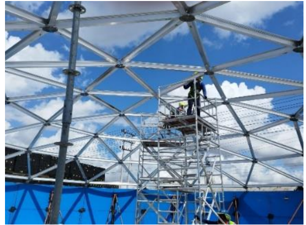
8. Installation of Dome Frame
