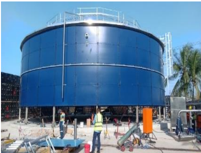
14. Lifting of Tank for 5 th Ring
