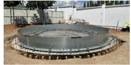
3. BSR Ring Installation - 1 st Tank
