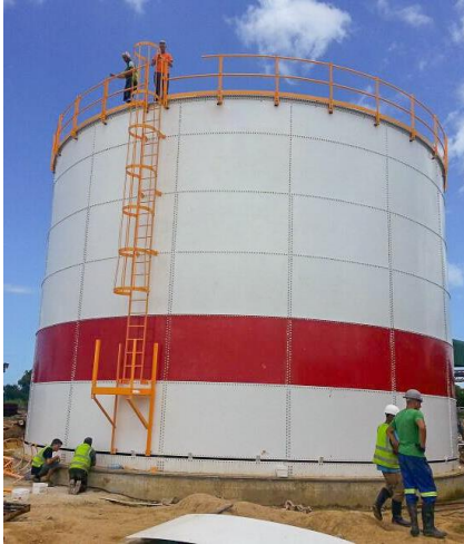
10. Installation of 6 th Ring
