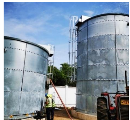
18. Installation of 6 th Ring
